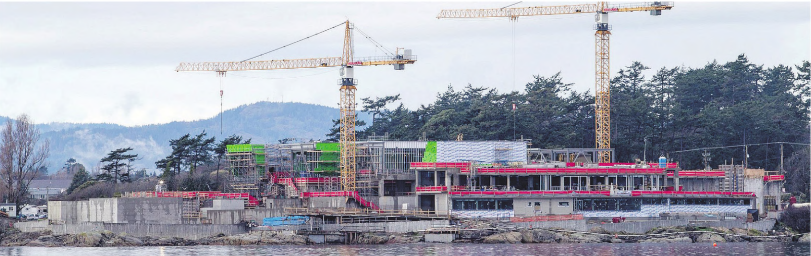
Biosolids will be a byproduct of the region’s sewage-treatment plant, under construction at McLoughlin Point. DARREN STONE, TIMES COLONIST
