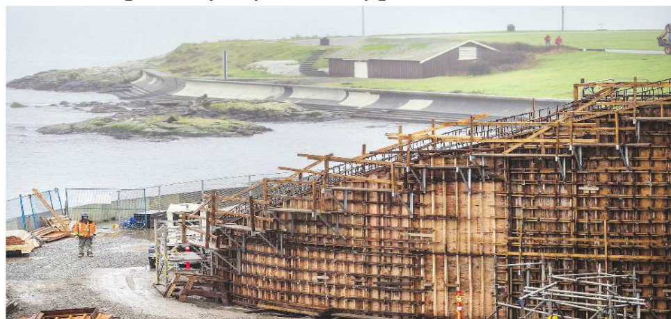
Crews work on expanding the Clover Point pump station, due to be completed in the middle of this year. DARREN STONE, TIMES COLONIST
