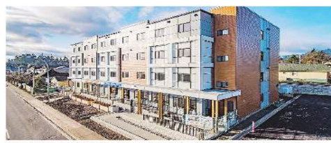
Samaritan Place supportive housing facility's residents were temporarily displaced following a mattress fire on Sunday. VIA B.C. HOUSING
